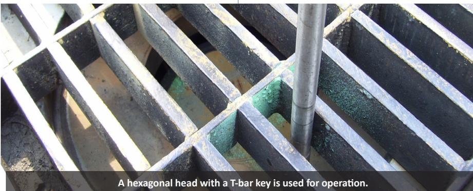
A hexagonal head with a T-bar key is used for operation.
